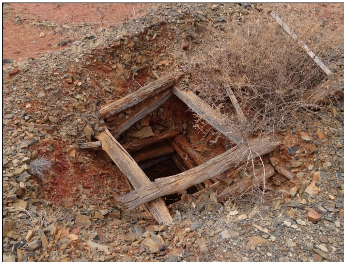
Figure 14: The framework around a possible mine shaft entrance. ID431.
