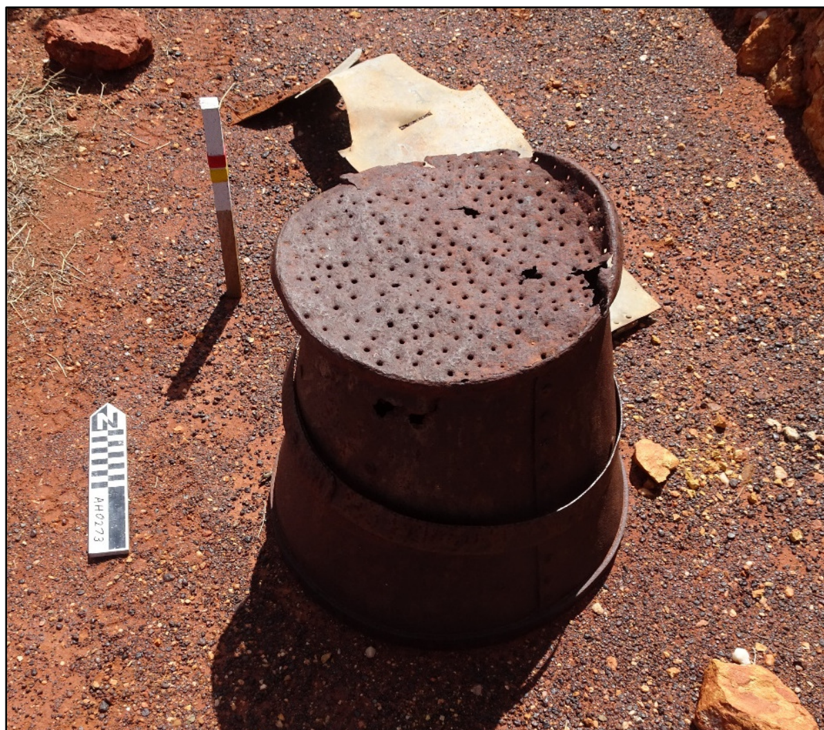
Figure 54: The air inlet at Afghan hut, formed by a perforated, inverted iron bucket. ID739.
