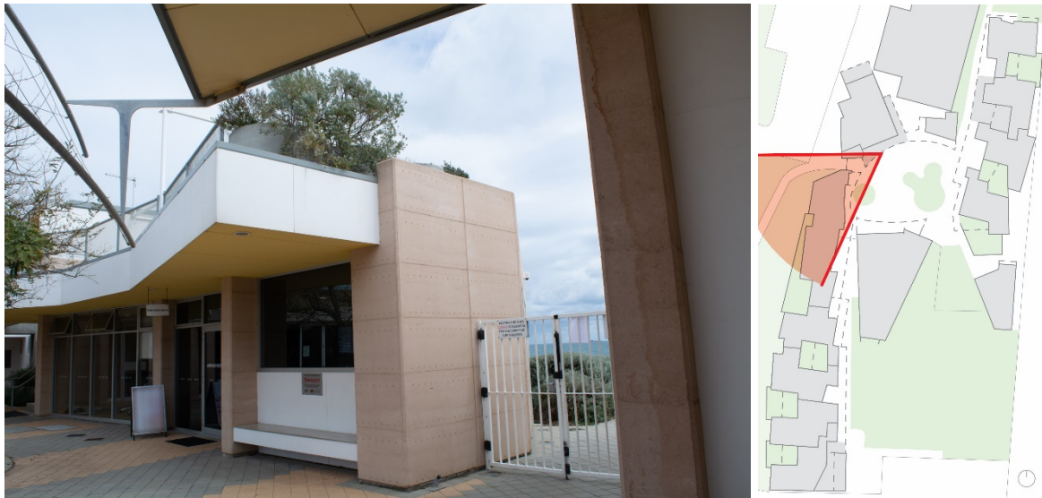
Figure 5.3 Case study school rammed earth walls at the entrance.
