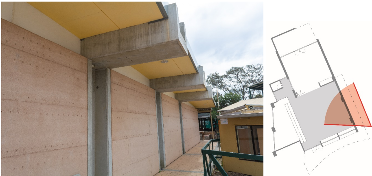
Figure 5.17 Upper primary observed classroom external gutters.
